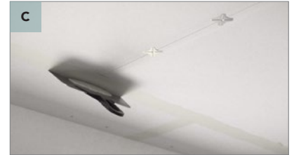
Fill joints, insert tape and finish joints: Use your preferred tool to fill the joint. Repeat until the joint is properly filled.
