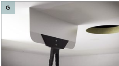
Check joints and center of panels.
